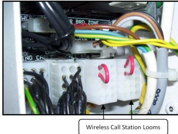
Figure 4: PSU PCB showing both Wireless Call Station Looms connected.
